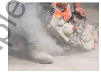
*Cutting concrete creates high levels of cement and silica dust*
