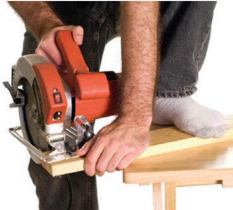
This worker is not using this equipment correctly and has therefore increased the potential for injury
