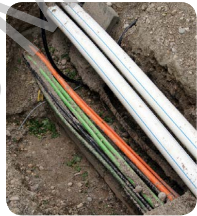
A shallow excavation revealing a collection of buried services
