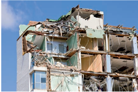
Explosions can cause severe damage
