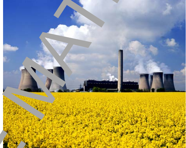
Possible source of environmental damage
